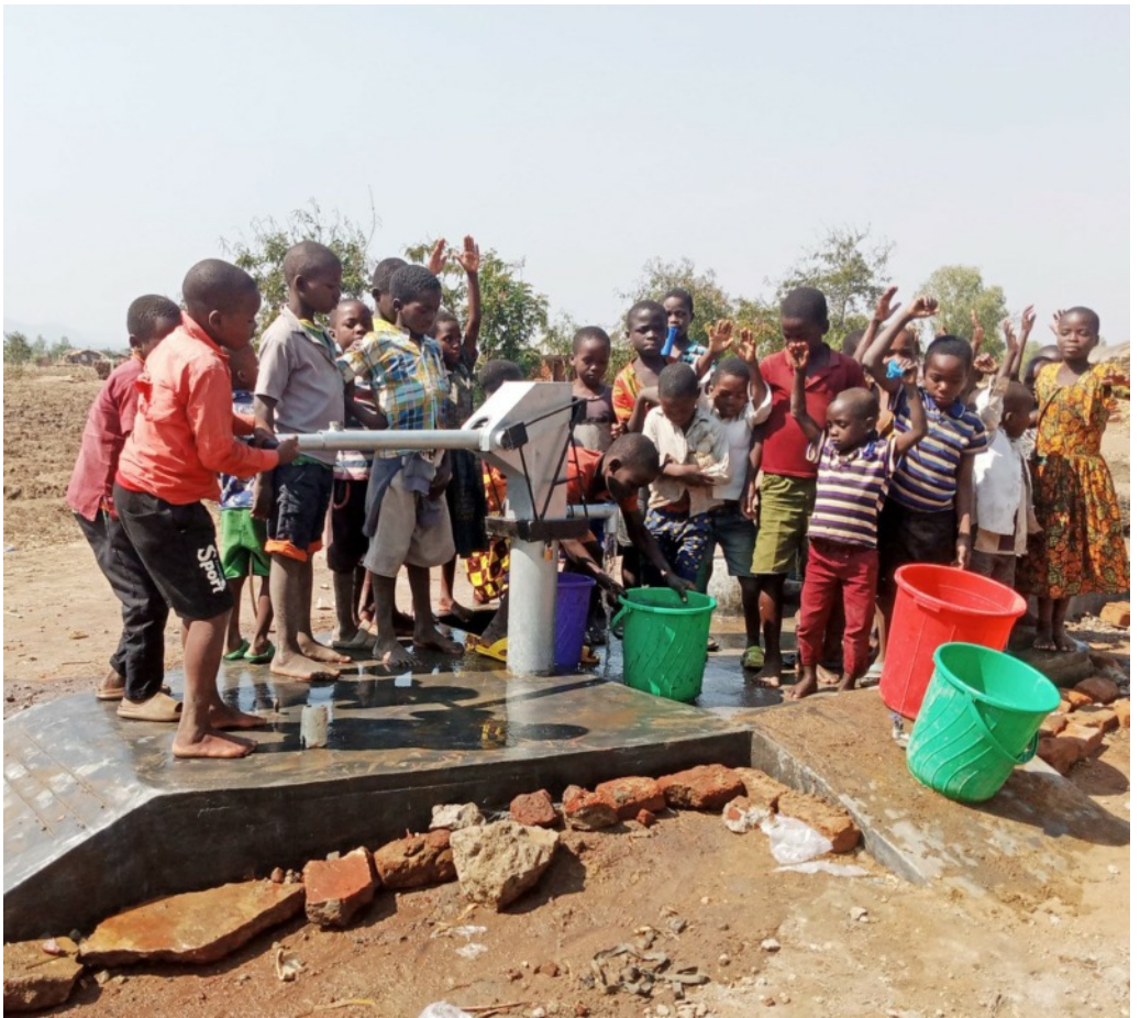
Pump at Mpoto School repaired! Project 374
